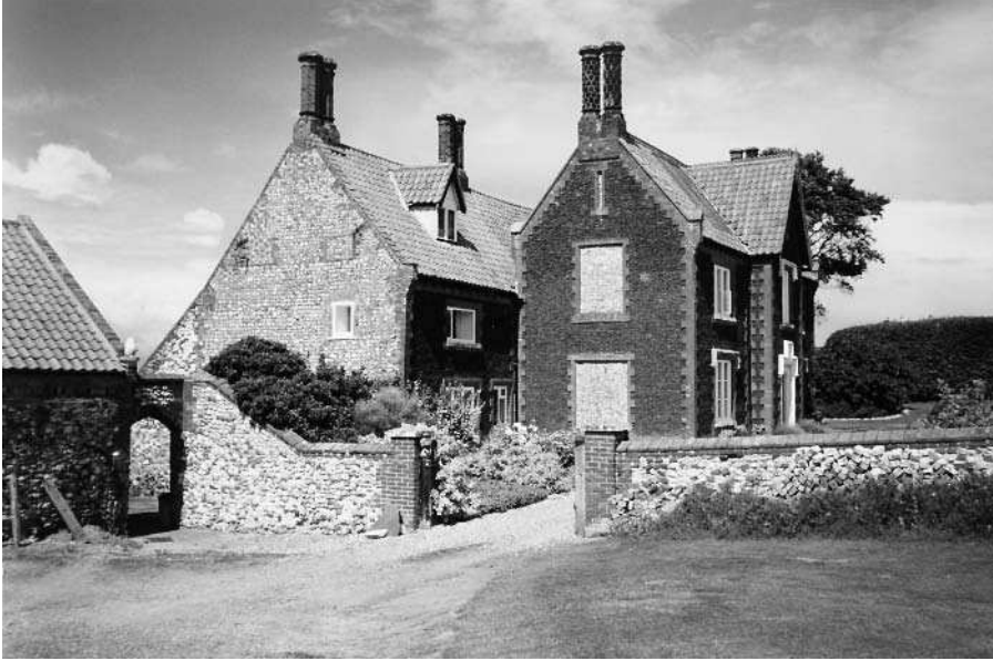
Plate 18: Choseley Manor, Norfolk, possibly the site of a preceptory of the order of St Lazarus. A nineteenth-century house (in the foreground) has been built up against an older structure, possibly with medieval origins.
